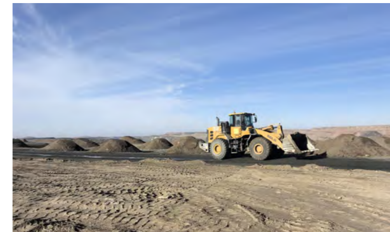
Ecological Restoration Construction
