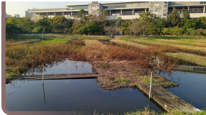
Ecological monitoring pathways built using retired timber sleepers to support habitat monitoring
