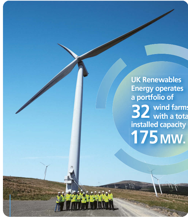
The Minnygap wind farm in Dumfries, Scotland, is one of 32 onshore wind farms operated by UK Renewables Energy.
