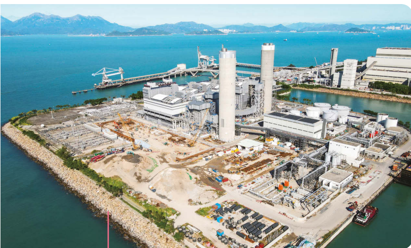
Aerial view of the L13 gas-fired generating unit at Lamma Power Station.
