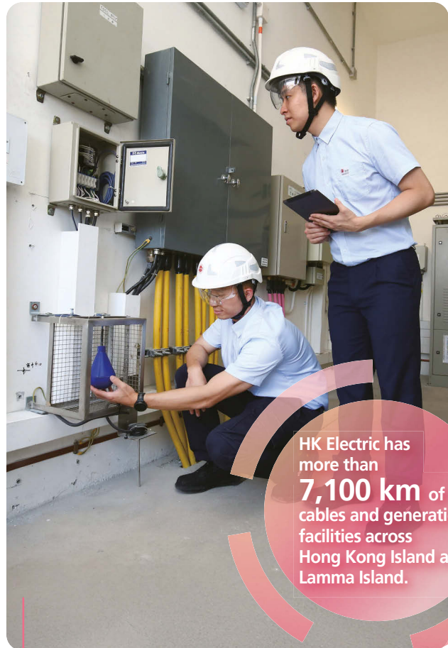
At HK Electric's Lamma Power Station, engineers inspect the resilience facilities such as this automatic water pump against flooding.
