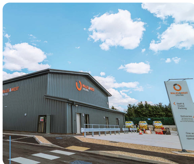
From its Cullompton depot in Devon, WWU crews carry out leak detection and repairs, pipework maintenance and replacement, and other routine upkeep to ensure the reliability of the regional gas network.
