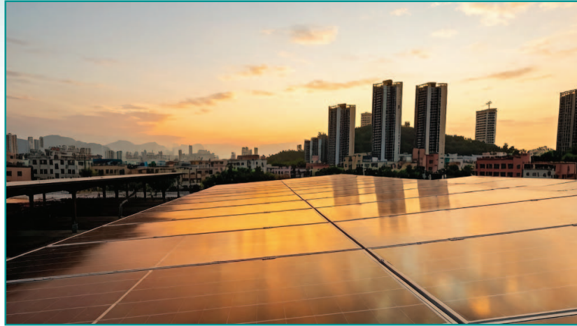
Solar panels are installed at our plant in Pingshan 坪山廠鋪設太陽能電池板
