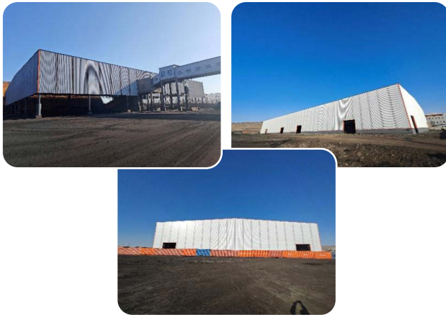
Three Newly Built Enclosed Coal Sheds in the Zhongqi Area
