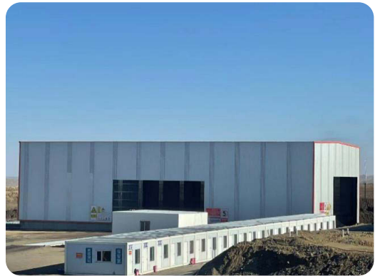
Newly Built Enclosed Coal Shed at Mandula Port
