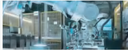
Digital and intelligent production workshop at the Hisense Hitachi Huangdao Factory
