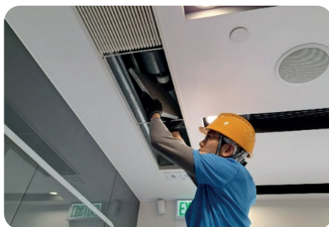
Maintenance of air ventilation systems
