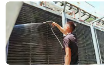
Air conditioning cooling tower cleaning
