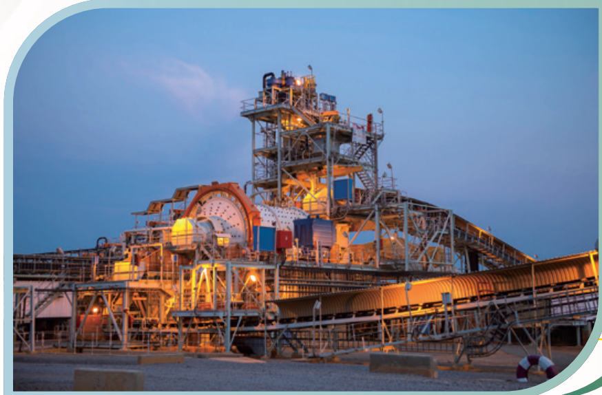
Kinsenda Mine - Processing Plant Kinsenda礦場 - 選礦廠
