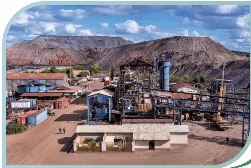
Ruashi Mine - Processing Plant Ruashi礦場 - 選礦廠
